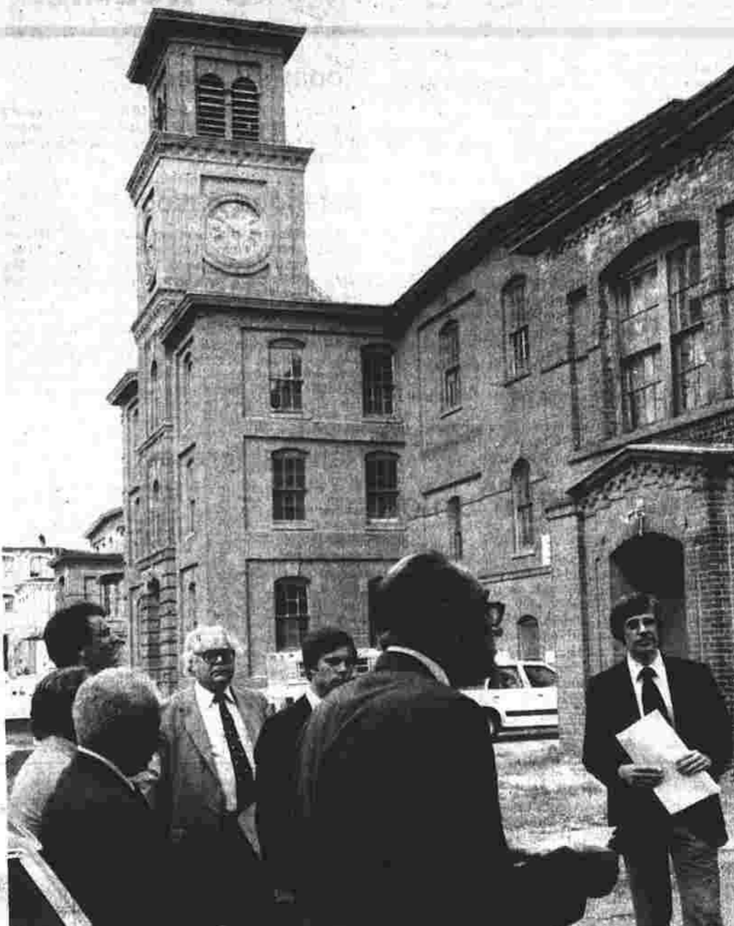
Mayor Stephen T. Penny, right, discusses plans for the renovation of the Cheney Brothers Clocktower Mill into apartments at a press conference held in front of the mill Friday. Attending the conference were town officials, building owners and architects and developers working on the project.
